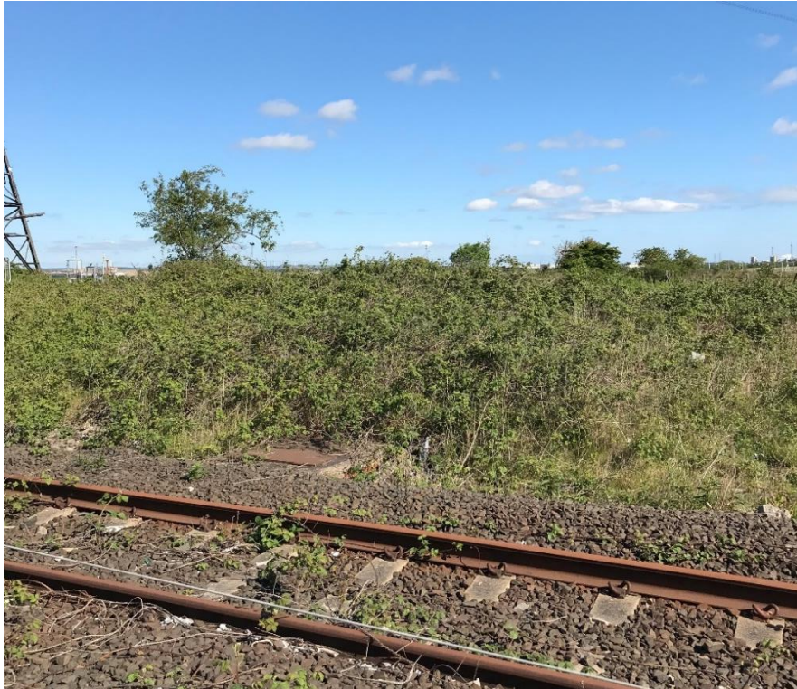
Photograph 31. Bramble scrub adjacent to disused railway
